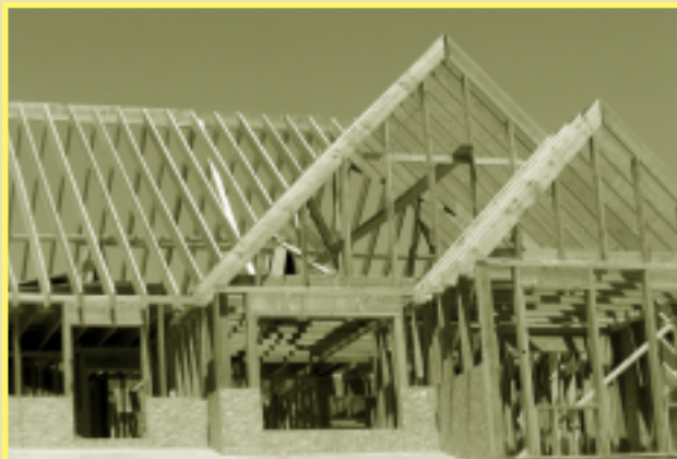
Figure 2. — Wood framing dominates single-family home construction in the United States.
